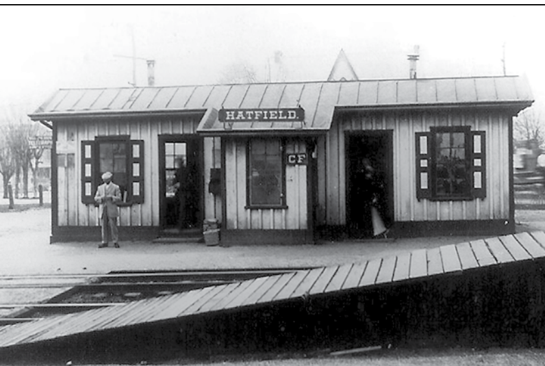
The original Hatfield Train Station, previously at the Cowpath Road crossing.
