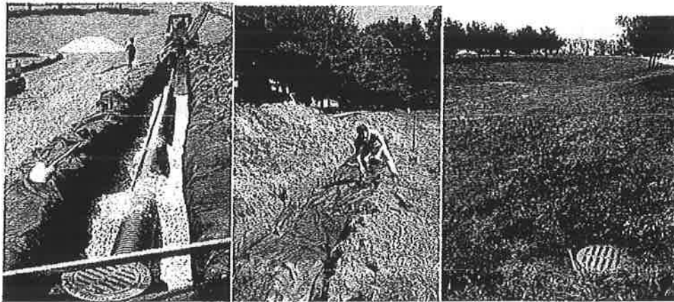
Figure 4: Example of Infiltration Trench Installation
