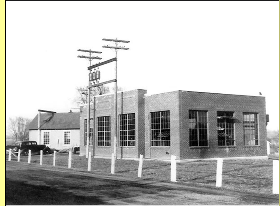
Electric Plant, Chestnut & S. Main Streets picture courtesy of the HMHS
