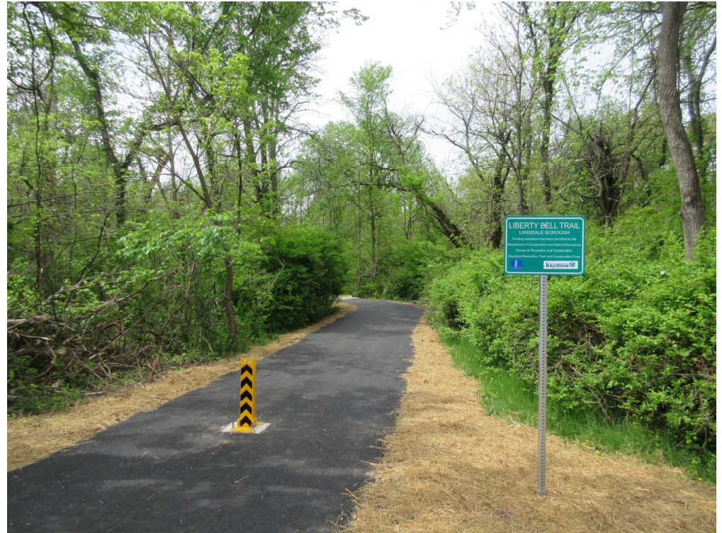
Photo of existing Liberty Bell Trail in Stony Creek Park.
