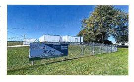
RICE (reciprocating internal combustion engine) Peaking installation. This consisted of 5.4 mw of peak shaving diesel generators. The project is expected to be commissioned COD (commercial operation date) on November 1, 2021. Ephrata is the first of nine Rice Peaking projects to come online in partnership with AMP. The other Pennsylvania participants include Perkasie, Hatfield, Schuylkill Haven, Mifflinburg, Quakertown Blakely, Weatherly and Girard."
